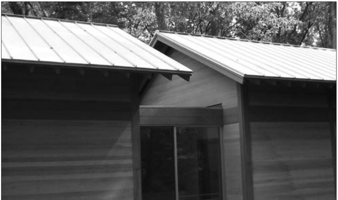
Standing seam Galvalume snap-lock panel
