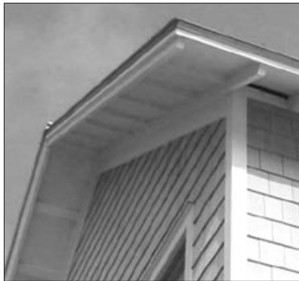
ALLOWED - EXPOSED RAFTER TAIL EAVE
