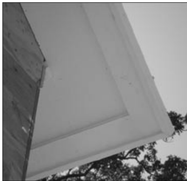
ALLOWED - DOUBLE PLYWOOD EAVE
