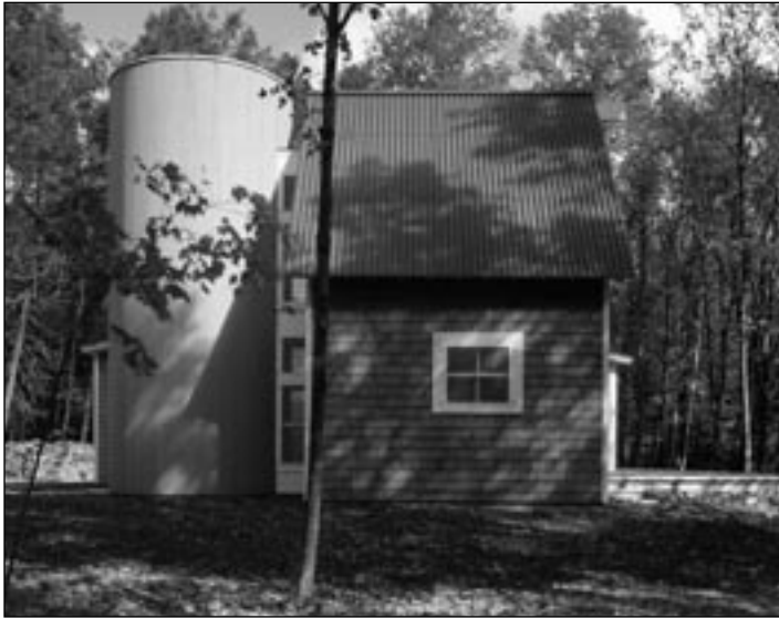
Corrugated Galvalume panel (min. 1" deep groove)
